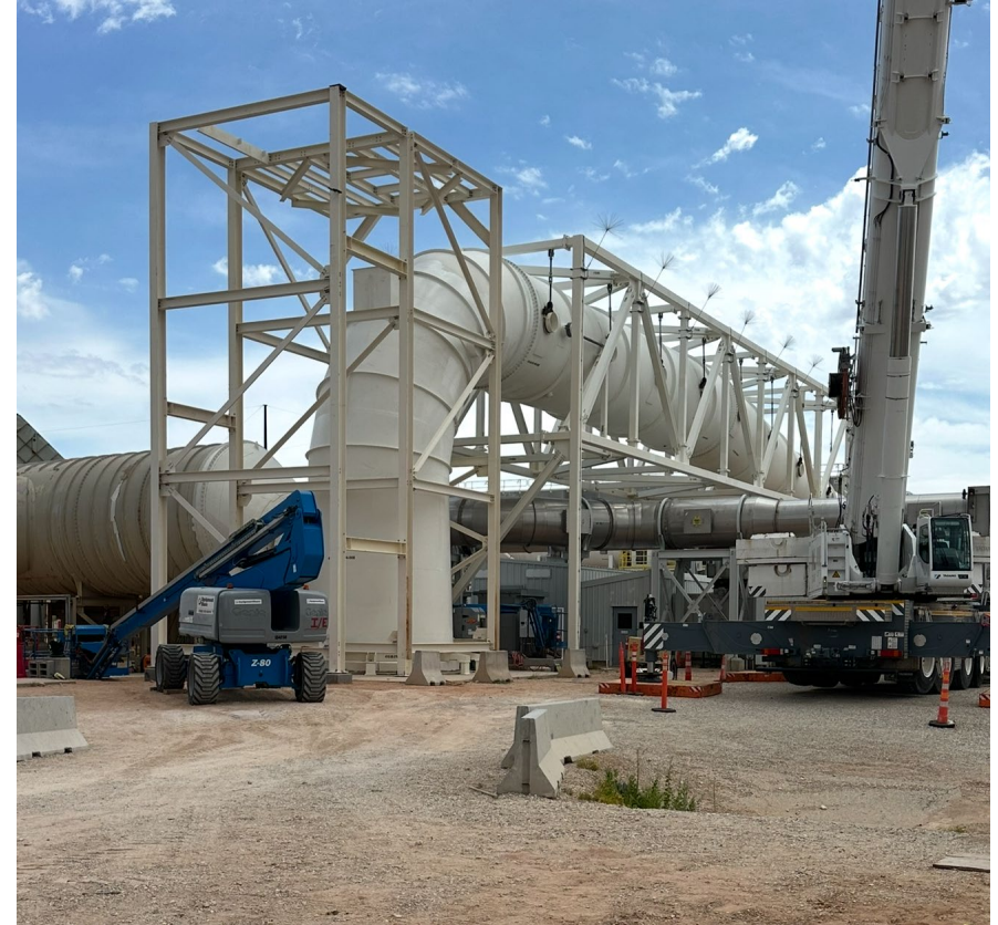
Completed exhaust shaft ductwork and support structure taking air to the new UVS.
