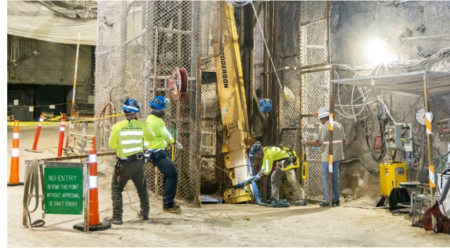
Work begins in the WIPP underground to refurbish the salt loading pocket infrastructure
