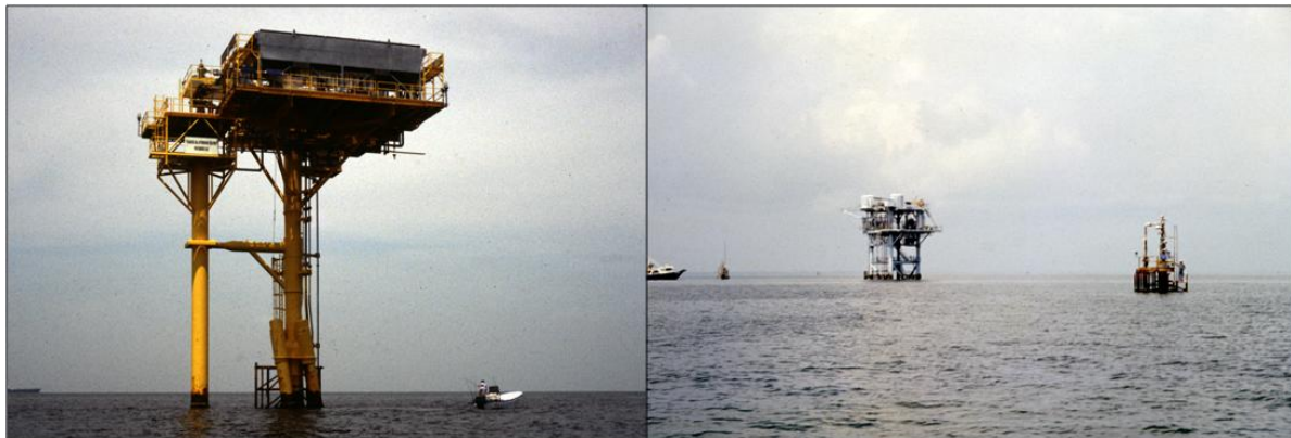
Figure 12. Platform in the open waters of the Gulf of Mexico off the Alabama coast (left) and wellhead (note the person on the wellhead for scale) and smaller platform are in the protected waters off the coast of Alabama (right) (Courtesy: Jack Moody, Mississippi).
