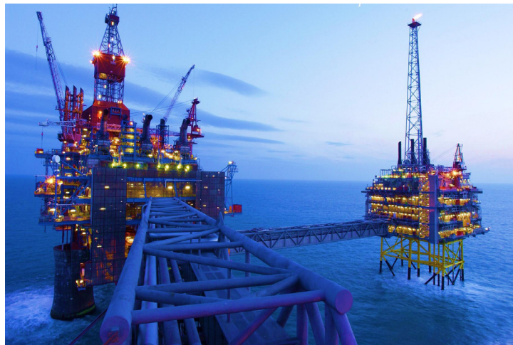
Figure 7. Photograph of the Sleipner production platform of the North Sea shelf, which hosts the first commercial CO 2 geologic storage project (Source: Statoil). 222
