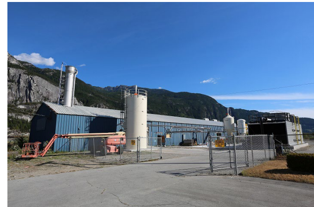
Carbon Engineering's research pilot facility in Squamish, BC
