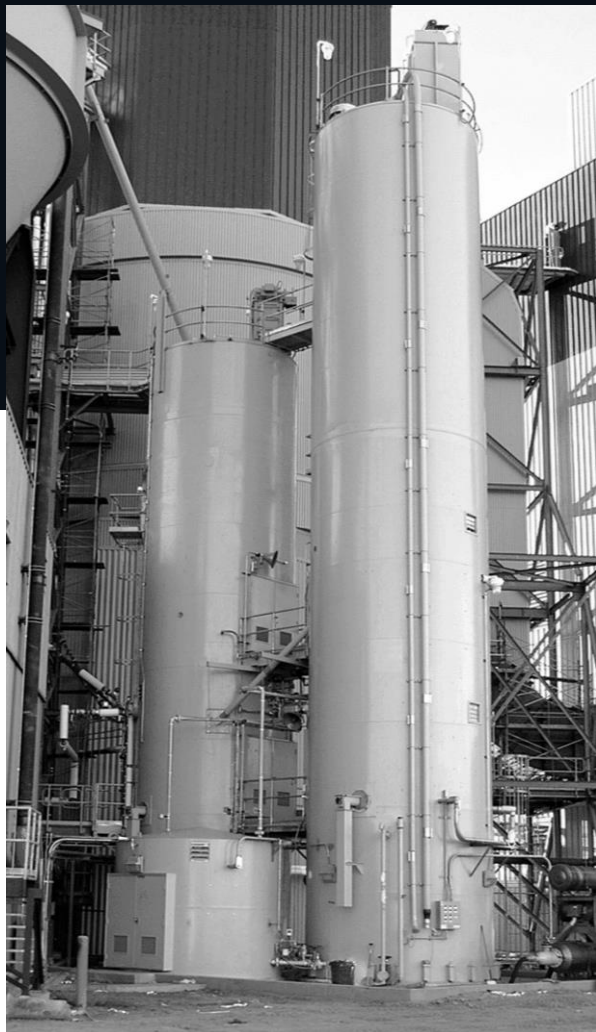
Back End SB sorbent system injected to ensure maximum mercury capture
