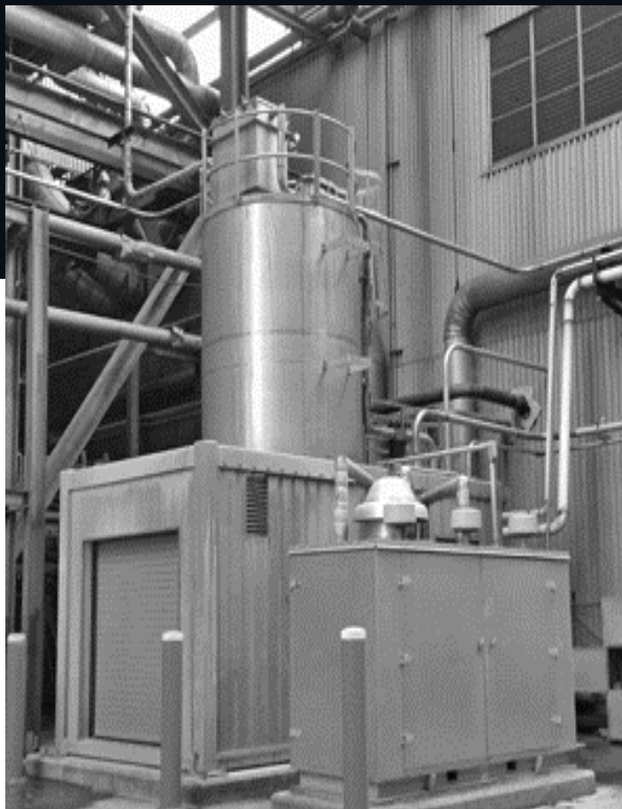
Front End SF injected directly into the boiler in minimal amounts.
