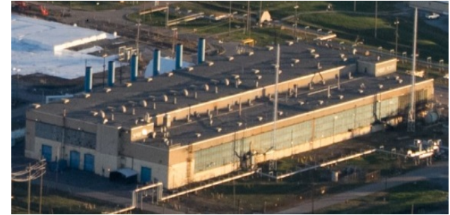
C-400 Cleaning Building
