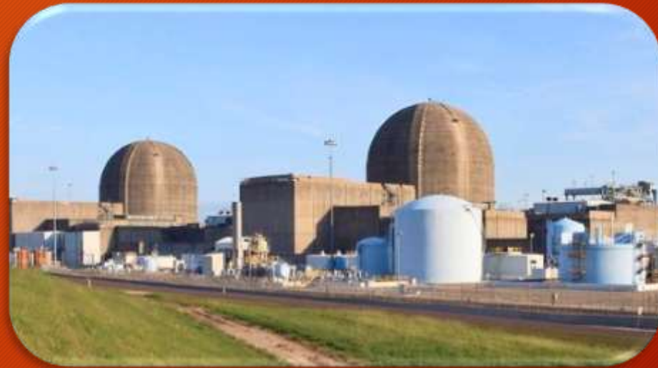
South Texas Nuclear Power Plant
