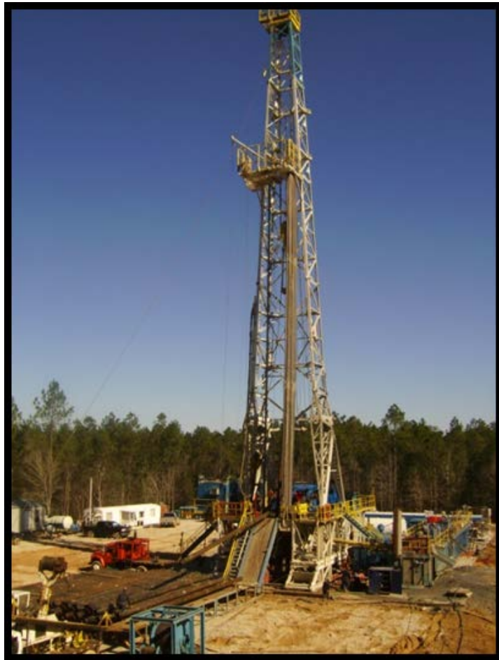
Installation of Injection Well D9-7 #2
