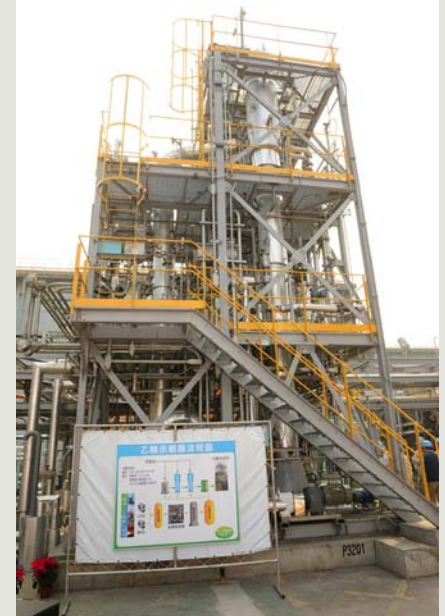
China Steel Corporation ethanol plant Feed gas: CO 2 +CO+H 2 Blast furnace gas (BFG), basic oxygen furnace gas
