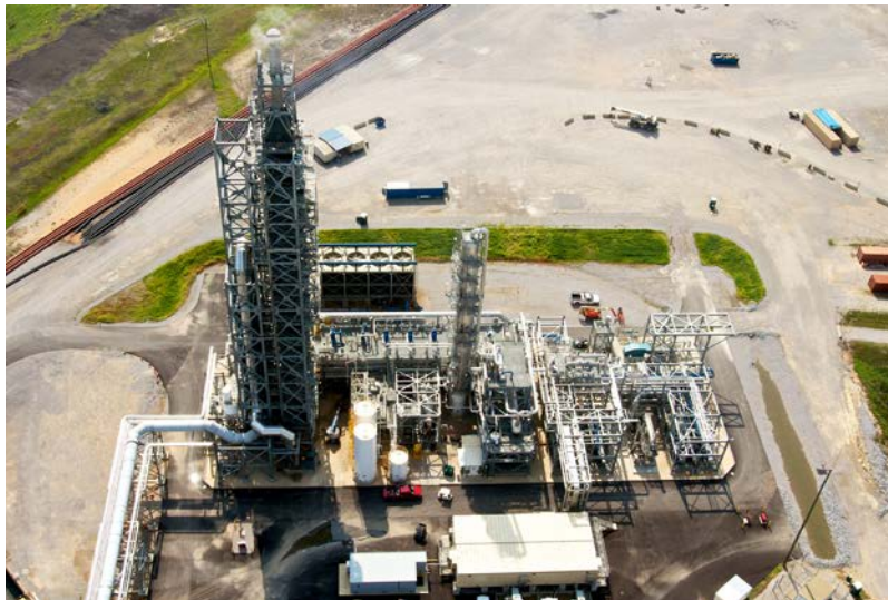
Figure 8. A photograph of the 25 MW CO 2 capture facility at Alabama Power's James M. Barry Electric Generating Plant located in Bucks, Alabama. CO 2 is captured using Mitsubishi Heavy Industries Ltd. Technology KM-CDR™, which uses an advanced amine solvent, and compressed for pipeline transport to support a SECARB CCS project in Citronelle, Alabama. (Source: Alabama Power, a subsidiary of Southern Company)
