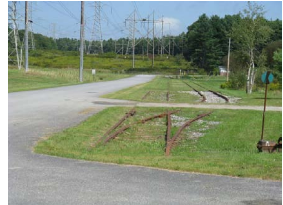
Current Condition of Onsite Rails at Maine Yankee
