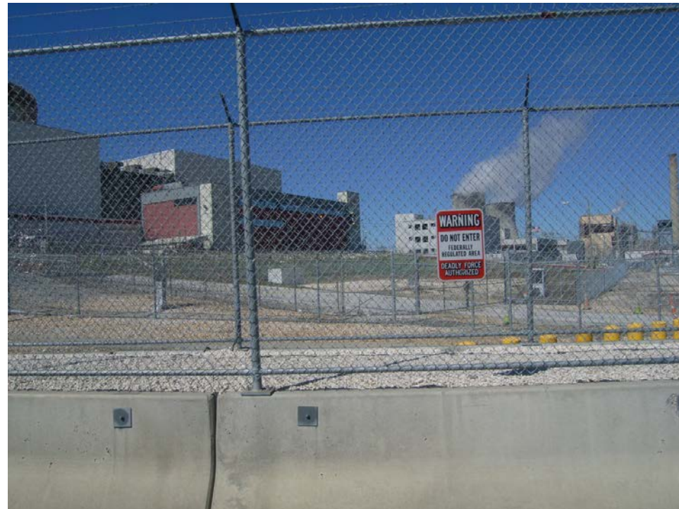
Future ISFSI Location (Looking North)
