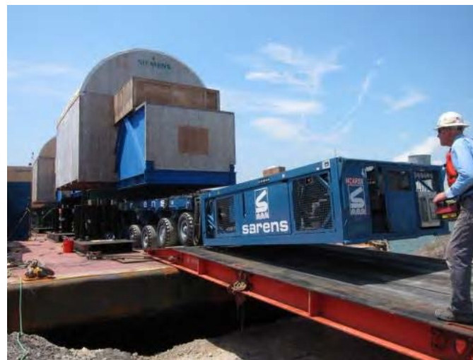
Turbine Components Being Unloaded Using Self-Propelled Modular Transporter (SPMT)
