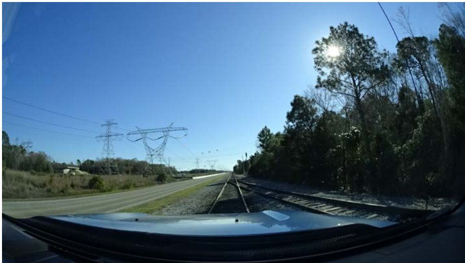
Onsite Industrial Spur at Cool Loop Junction
