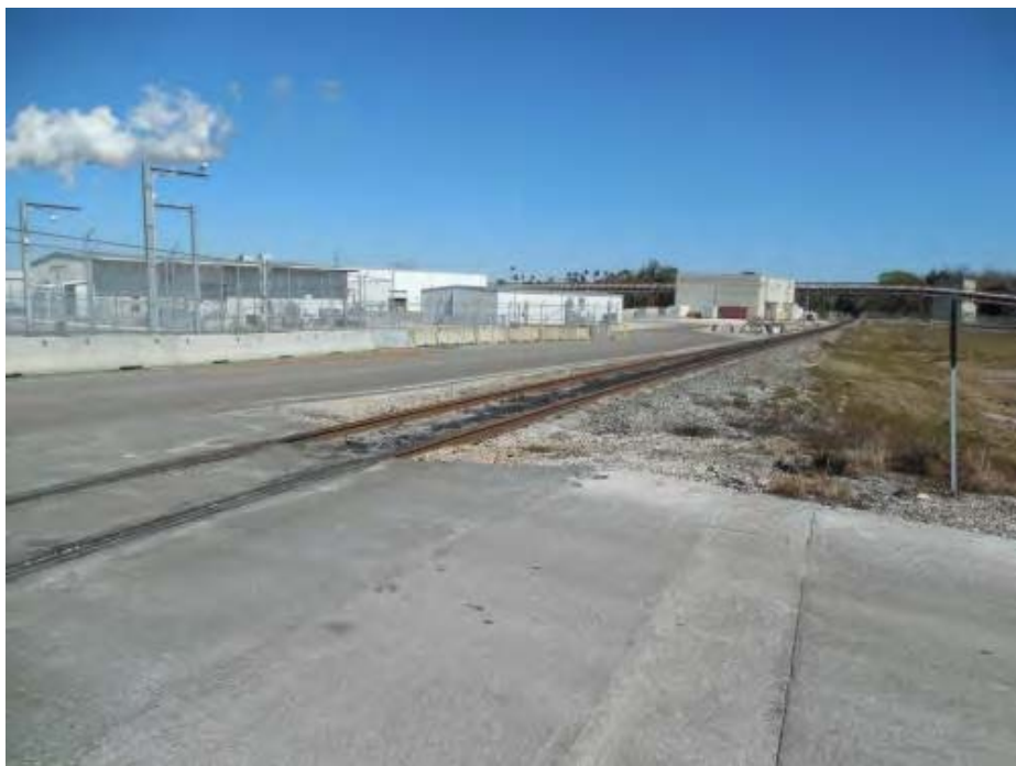
Onsite Rail Facing East
