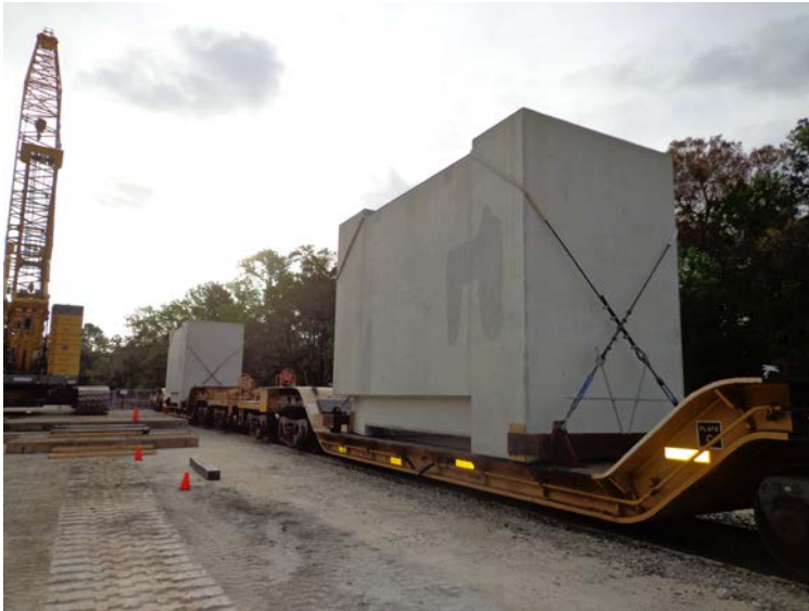
Two Horizontal Storage Modules Loaded onto Railcars
