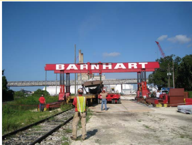
Unloading Generator Rotor
