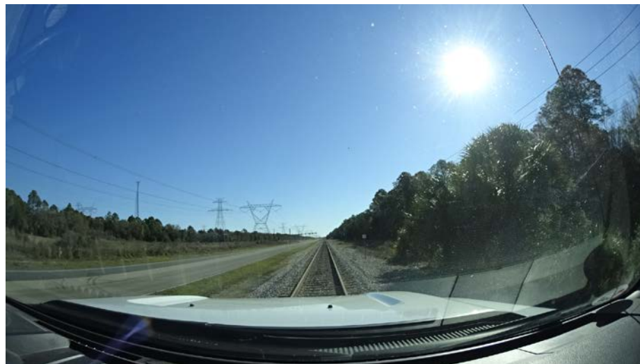
Onsite Industrial Spur Approaching US Highway 19 from the West
