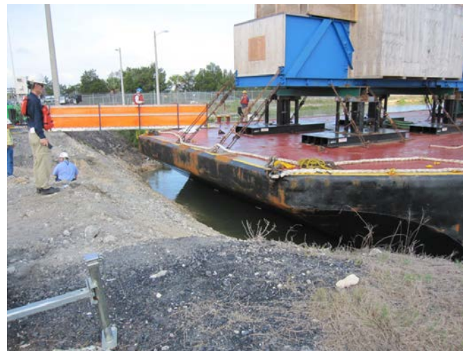
Docking Barge with Turbine Components
