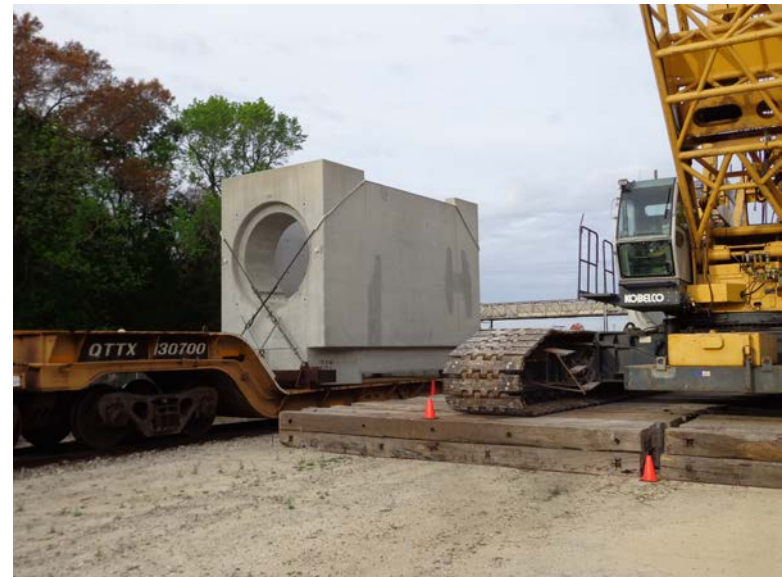
Horizontal Storage module Staged for Unloading
