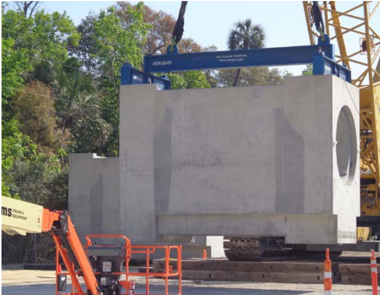
Horizontal Storage Module Being Unloaded from Railcar
