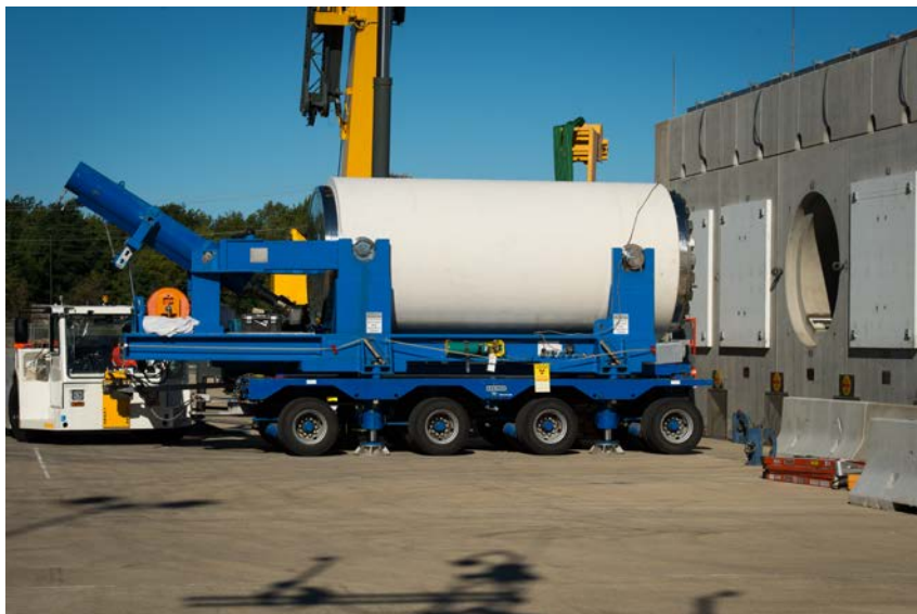
Photos courtesy of AREVA TN
