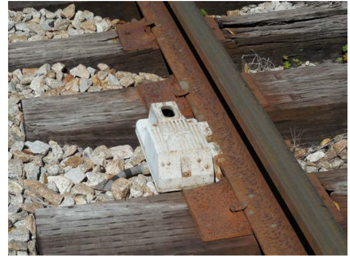
Hot Bearing Detector
