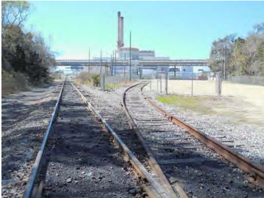
Junction of Onsite Industrial Spur and Nuclear Spur
