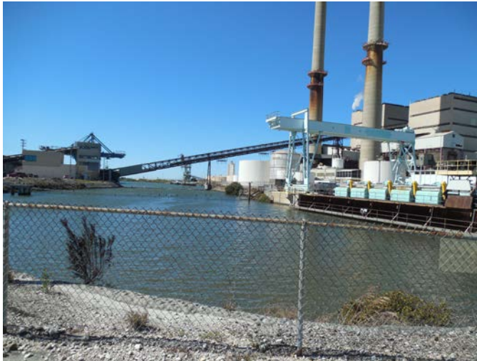
Coal Barge Unloading Area (Left) and Coal Conveyor
