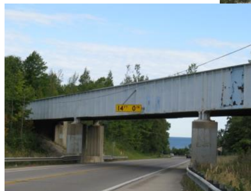
Low Overhead Bridge Near Big Rock Point
