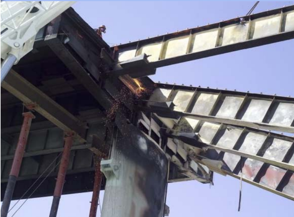
Girder cutting after concrete removal
